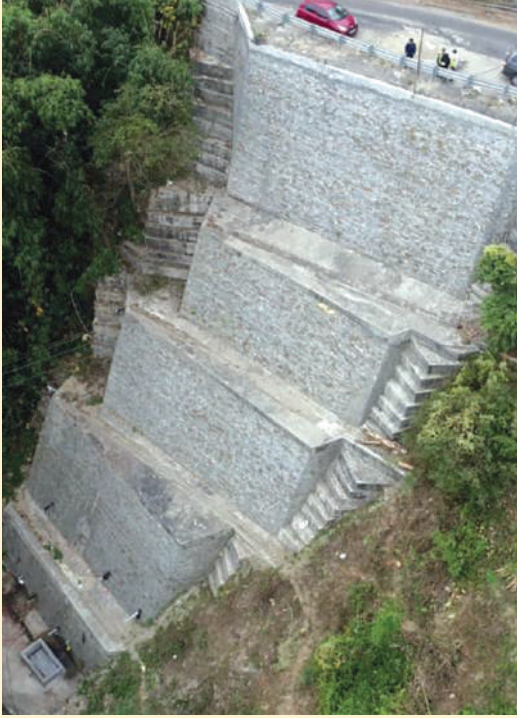
(Picture 10: After restoration, S1 spot, RE structure of 34.9 Mt.)
