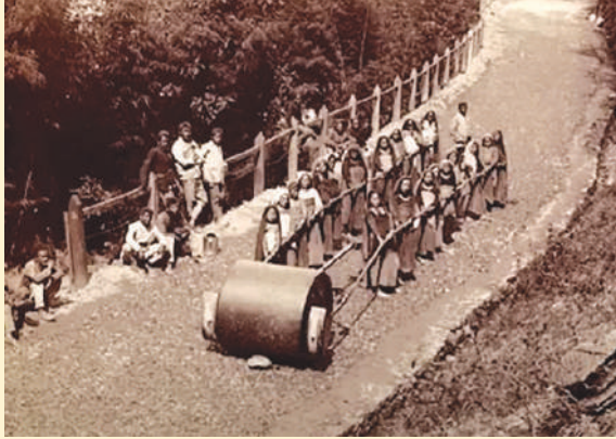
(Picture 2: The construction of Hill Cart Road).
