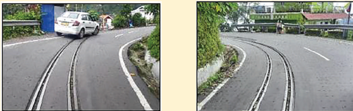
(Picture 19: Railway track crossing the National Highway at-grade)
