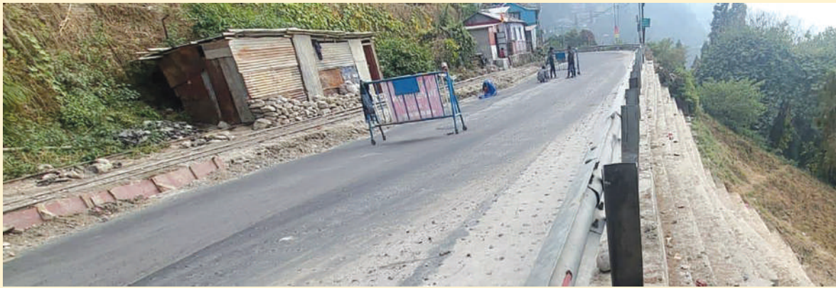
(Picture 15: Photo of the same spot after restoration)
