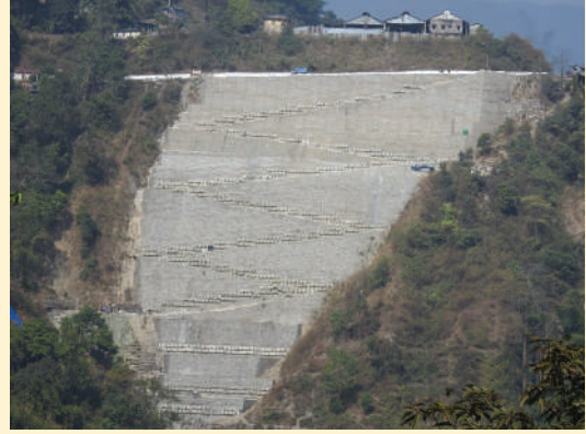
(Picture 11: After restoration, S2 spot with RE structure height of 102.8 Mt, highest in the world.)
