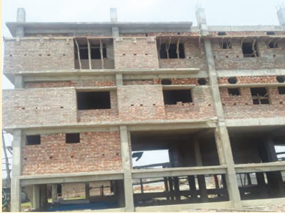
Fig- 4: Mandarmani MPCS of Purba Medinipur under construction
