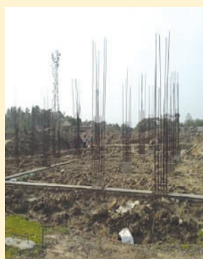
Fig-5: Excavation of earth during construction work at Chaital
