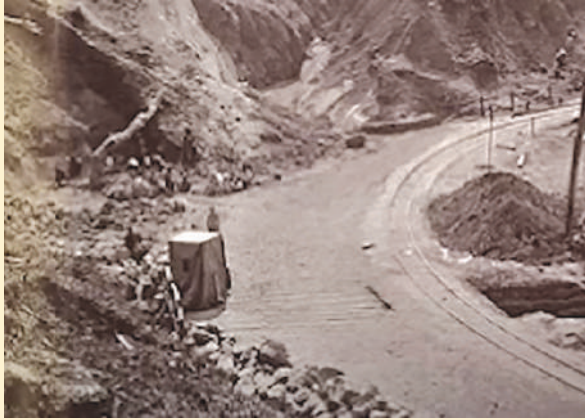
(Picture 5: Laying of railway track by the side of Hill Cart Road)
