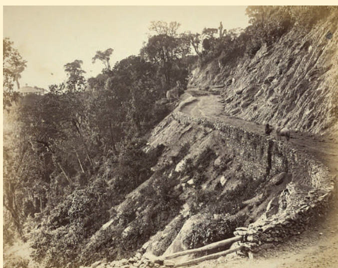
(Picture 1: Construction of the metalled Darjeeling Hill Road connecting Darjeeling to Siliguri shown at the half-way point at Kurseong, 19 and half miles away from Darjeeling).
